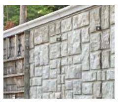
The all-aluminum ashlar stone concrete form uses an advanced stamping method that allows the aluminum sheet to be stamped in a deep ashlar-stone pattern. The result is a natural looking ashlar pattern without the need for formliners. The ashlar stone forms are compatible with any aluminum forming system. www.wallties.com
